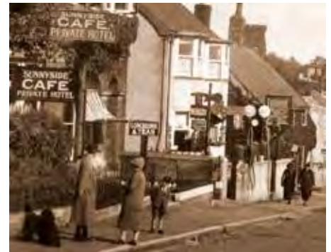
7. Woolards Garage in 1925 with its petrol pumps
