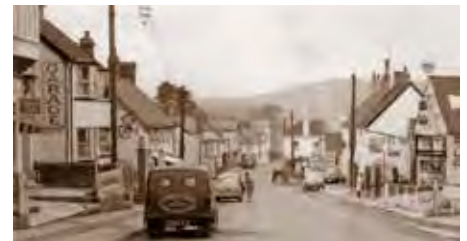
8. 1953 photo of the two garages opposite each other.
